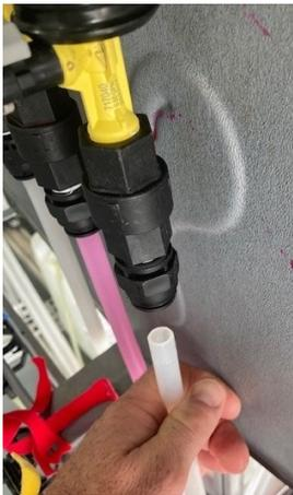
2. Install a bare 2-4 foot hose and point toward a drain or a bucket.
